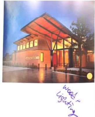
Exterior entrance - Wood & lighting
